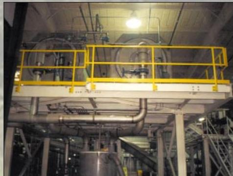
Two MDS units in secondary (waste activated) sludge thickening service. Feed of <1% is pretreated with polymer at about 6 to 9 kg/ton of dry solids.
